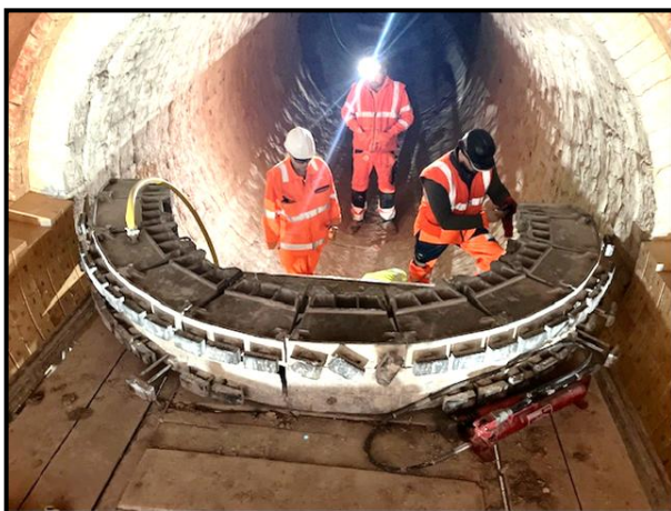
Toppled Frame inside Rotary Kiln
