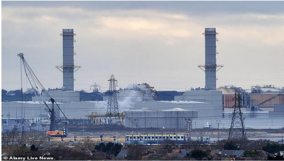
Fig 3; picture of Isle of Grain power station chimney collapse in Storm Eunice in 2022. Source: 54379881-10530003-A chimney has collapsed at a Power Plant on the Isle of Grain in-m-68 1645261658002.jpg (634x495) (dailymail.co.uk)
