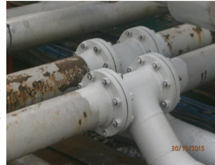
Tank 53 and 54 tie-ins
